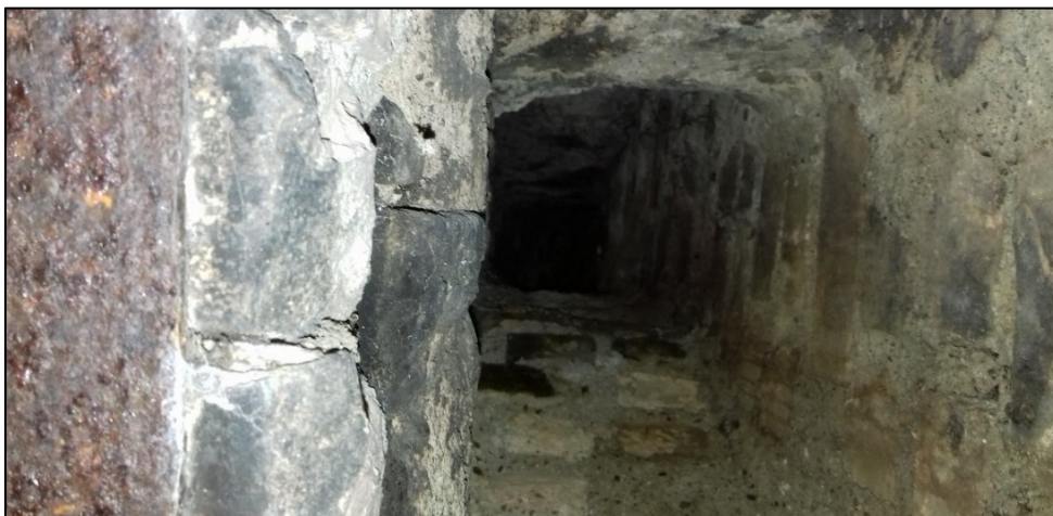
Plate 1. Abandoned gate lodge showing examples of potential roost spaces.
